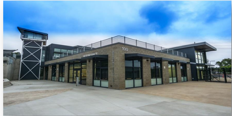
EWMS – Campus Re-Construction
